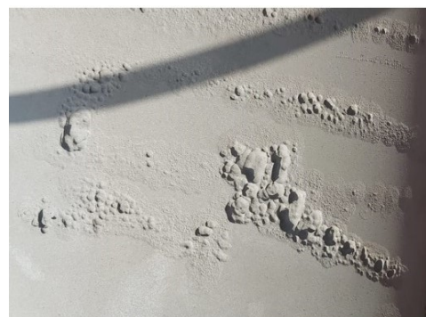
Figure 3. Cylinder casing localized pitting.
